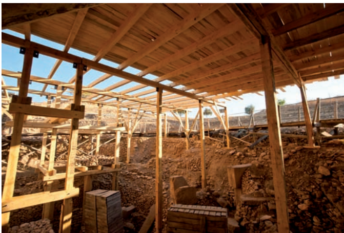
The wooden shelter during construction (Photo: NB).
