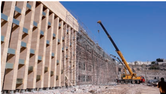
Construction work at the new museum in winter 2013 (Photo, top: NB, bottom: MA).
