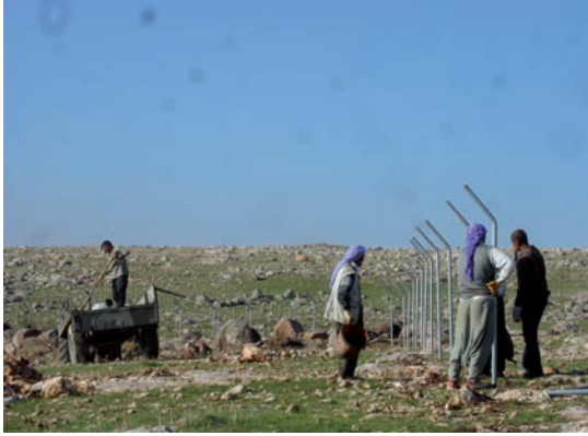
A group of the excavation workmen erecting the perimeter fence in winter 2012/2013 (Photo: MG).
