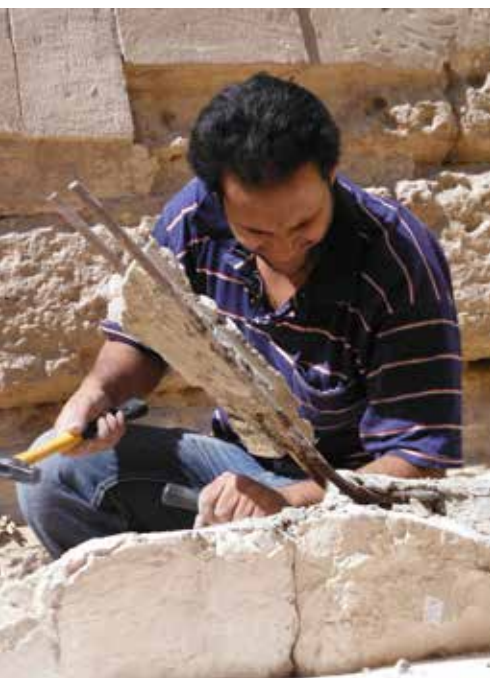
The old, damaged restoration with gypsum is removed by Mahmud Abu Seid, a team member trained by the project's conservator, E. Peintner
