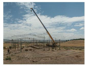
Setting the roof beams of the shelter construction with the help of a truck crane in October 2012.
